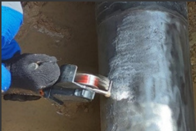
Fig. 1: Surface preparation on progress
