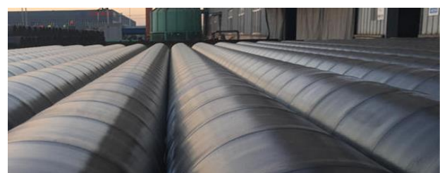
COATED PIPE AND IMPACT (PROTECTION)
