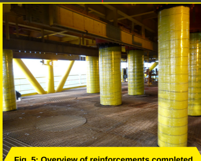
Fig. 5: Overview of reinforcements completed
