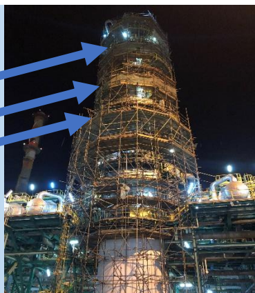
Fig. 1: Column overview with welds location
