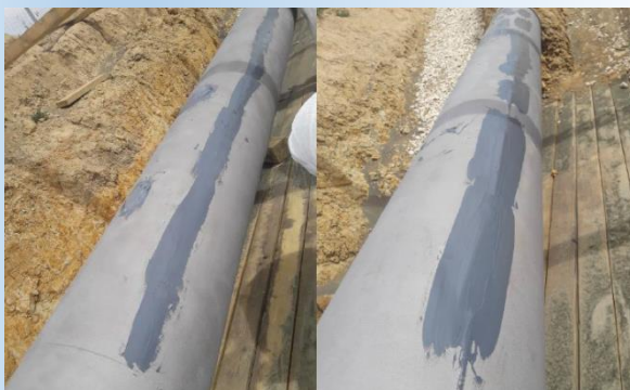
Fig. 2-3: Filler application over the defect area
