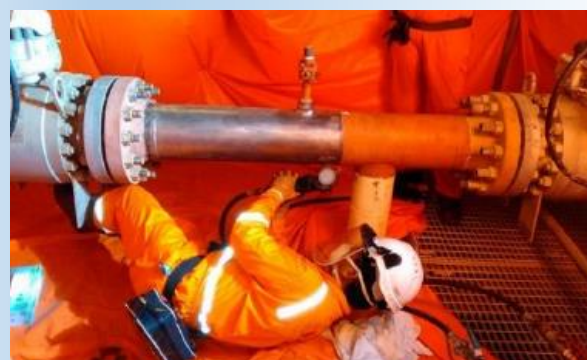
Figure 2: Surface preparation on progress using Bristle Blaster
