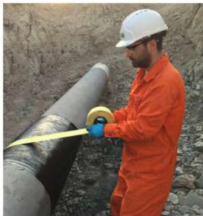
Figure 1. R4D wrapping in progress.
