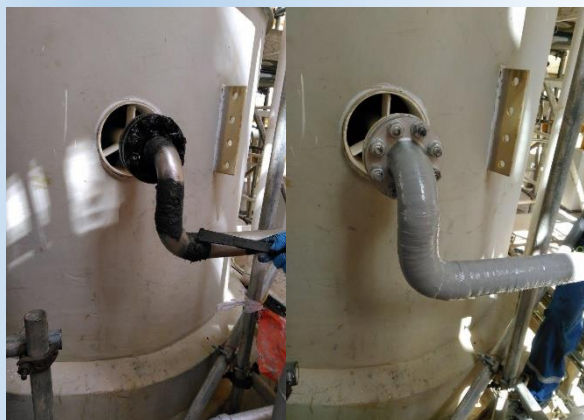
Fig. 1: Filler applied on defected joint area Fig. 2: Piping repaired with R4D
