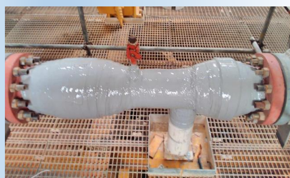
Figure 4: Repair overview (pipe spool A)
