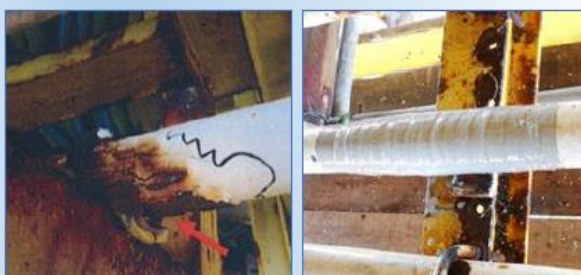
Fig. 5-6: Pipe on support reinforcement (before/after)
