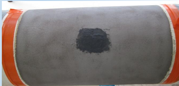
Fig. 2: View of the delimited repair area to be wrapped & Example of filler F3X8 application on 12" pipe defect
