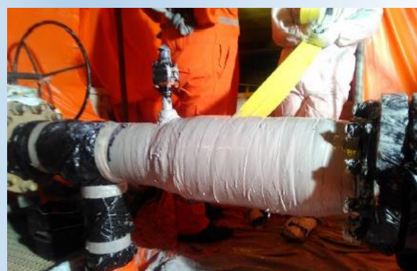
Figure 3: R4D composite wrapping on progress
