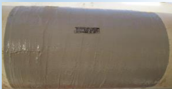
Fig. 4: Wrapping completed & Identity plate installed
