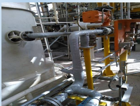
Fig. 3: Complex piping section repaired with R4D
