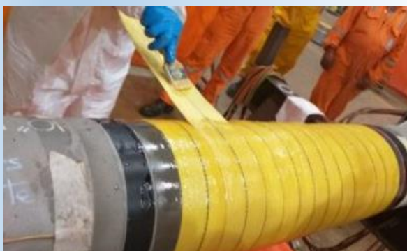
Figure 2: R4D composite wrapping in progress (step 3)
