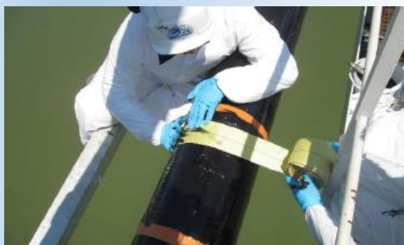
Fig. 3: Composite wrapping on progress
