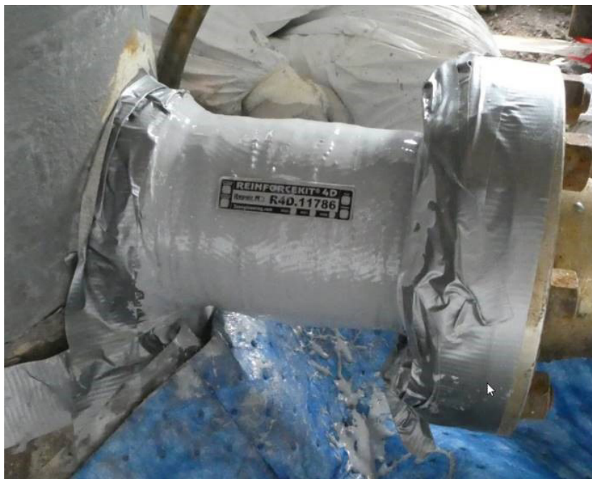
Figure 4. Repair overview with ID plate installed for traceability.
