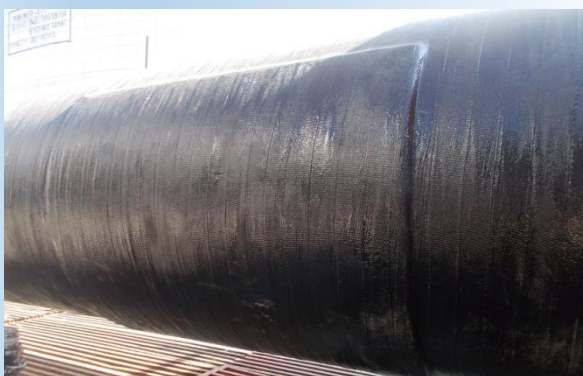
Fig. 2: Section of straight line with irregularity perfectly wrapped with R4D
