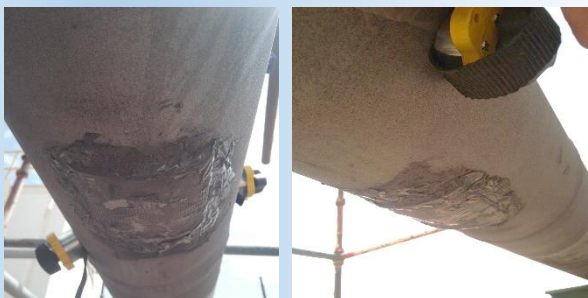
Fig. 2-3: Leak sealed with metallic plate and F3XS1
