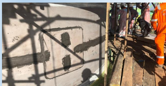
Fig. 2: F3XS1 application on weld
