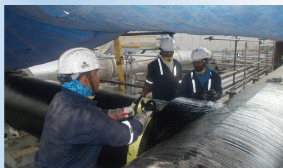
Fig. 4: Tee reinforcement – R4D wrapping on progress
