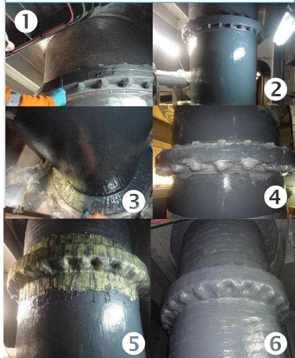
Composite repair steps
