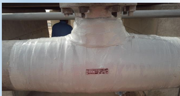
Fig. 6: Wrapping completed (12 layers) & ID plate installed
