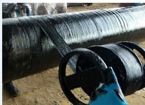
Figure 4: Composite wrapping on progress using specific handles
