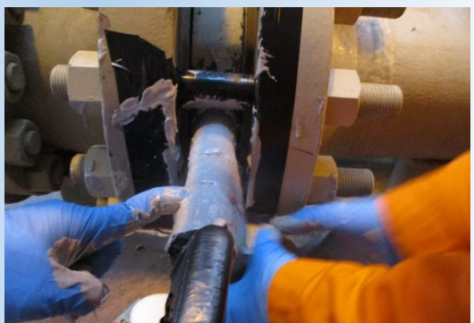
Fig. 3: Wrapping on progress
