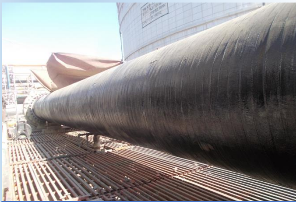
Fig. 1: Example of straight line wrapped with R4D
