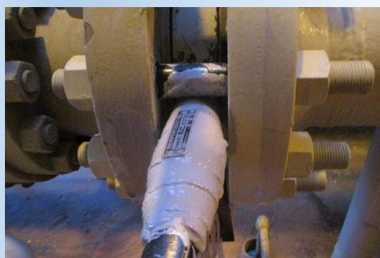
Fig. 4: Repair overview with ID plate
