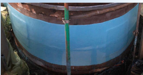
Fig. 6: Wrapping completed (4 layers)
