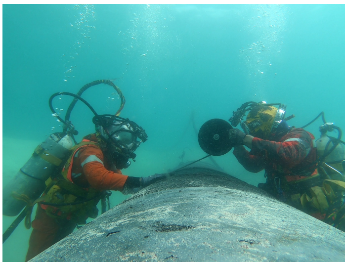
Figure 1. R4D composite repair wrapping in subsea environment.
