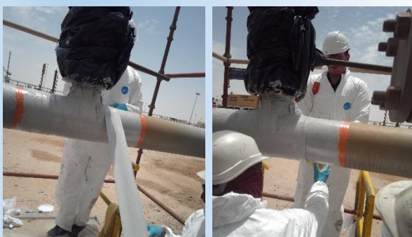
Fig. 4-5: Wrapping in progress
