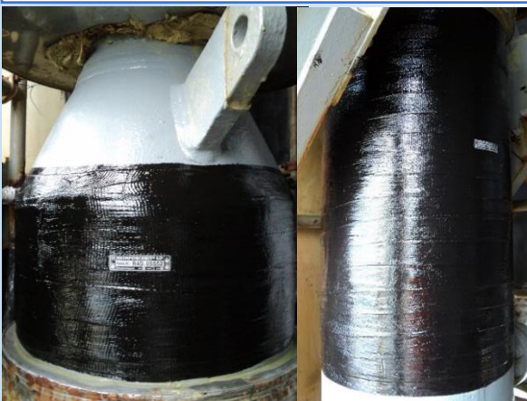
Figures 3 & 4: Composite wrappings finished on heat exchanger (2 defected areas)
