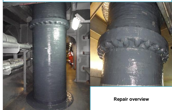
Composite repair steps
