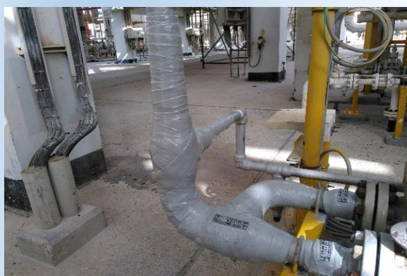
Fig. 4: Another complex piping repair overview completed with ID plate for traceability
