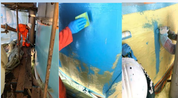
Fig. 3-4-5 : Wrapping in progress
