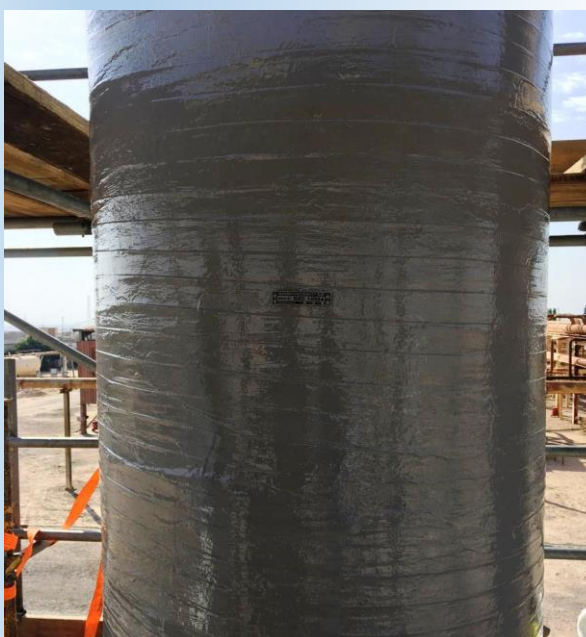
Fig. 4: Wrapping completed (6 layers) with ID plate
