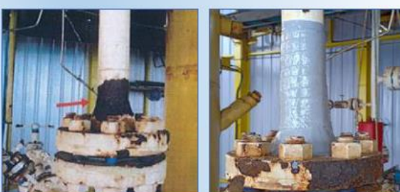
Fig. 7-8: Flange reinforcement (before/after)
