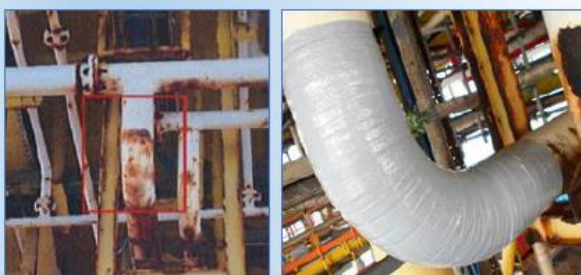
Fig. 3-4: Elbow reinforcement (before/after)
