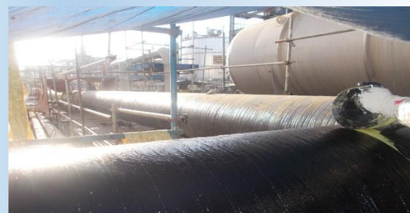
Fig. 3: Elbow reinforcement – R4D wrapping on progress
