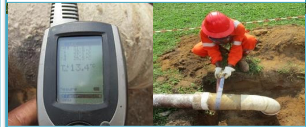
Climatic conditions measurements and surface preparation
