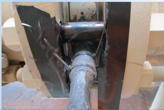
Fig. 2: Filler and bended plate applied on defected area
