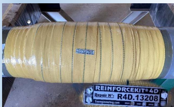
Figure 3: Repair overview with ID plate (step 4)
