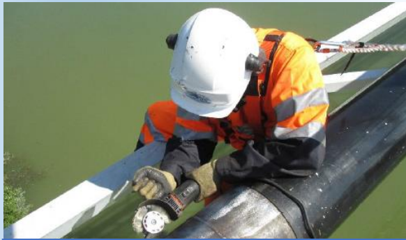
Fig. 1: Surface Preparation using Bristle Blaster®
