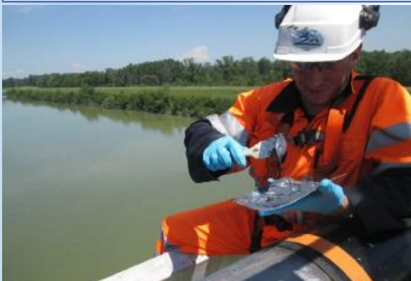
Fig. 2: F3X8 filler application
