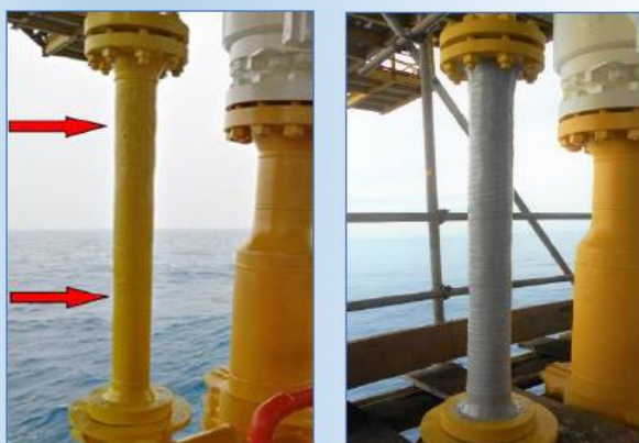
Fig. 1-2: Straight line reinforcement (before/after)
