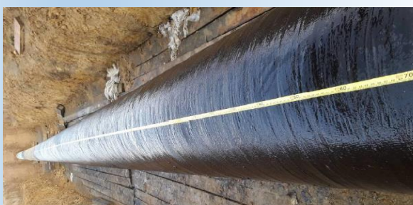
Fig. 6: Wrapping completed and measurement of the repair
