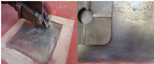
Fig. 1&2: Surface preparation on progress using Bristle Blaster
