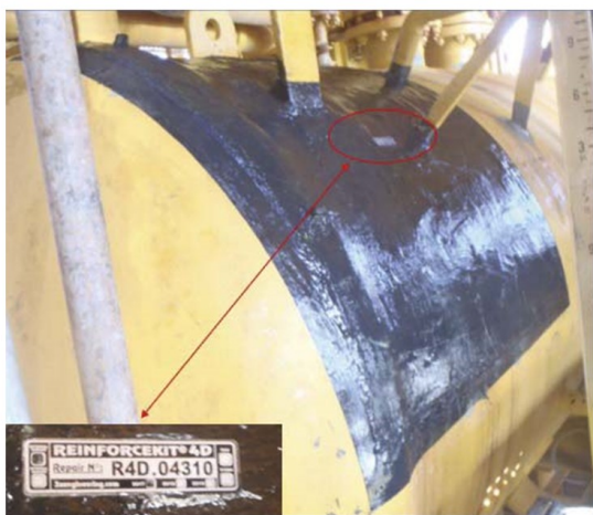
Figure 5. Final overview of the repair with ID plate.
