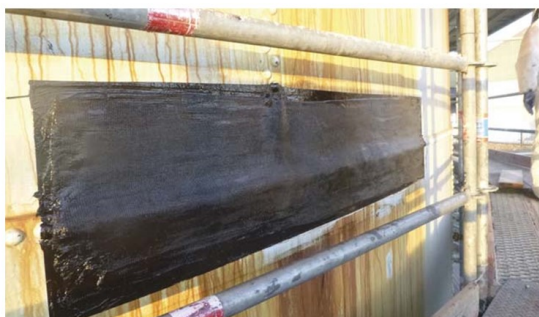
Figure 2. Example of REINFORCEKIT PATCH installed on water tank.
