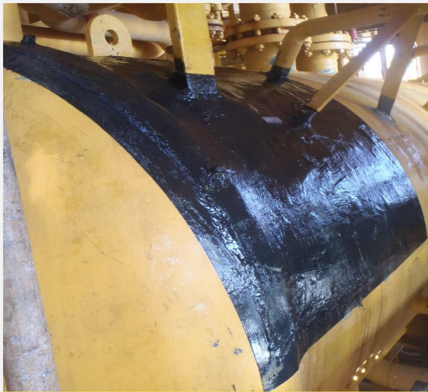
REINFORCEKIT® PATCH INSTALLED ON REBOILER (VIETNAM)
