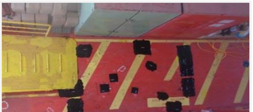
REINFORCEKIT® PATCH INSTALLED ON FPSO DECK (VIETNAM)
