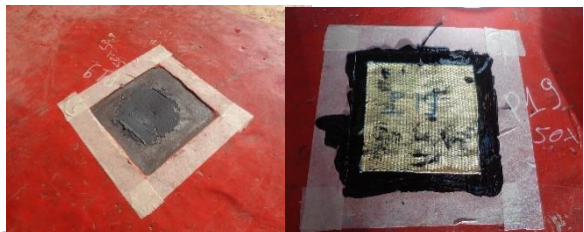
Fig. 3&4: F3X8 filler and R3X55 resin applications
