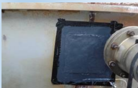
Fig. 5: Composite patching completed (5 layers)
