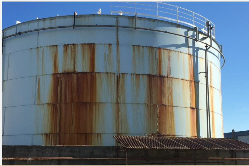
TANK TO BE REPAIRED – GENERAL VIEW
