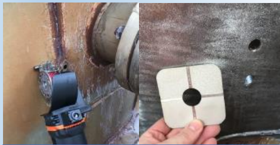
Fig. 2 & 3: Surface preparation in progress using Bristle Blaster® & roughness checking
