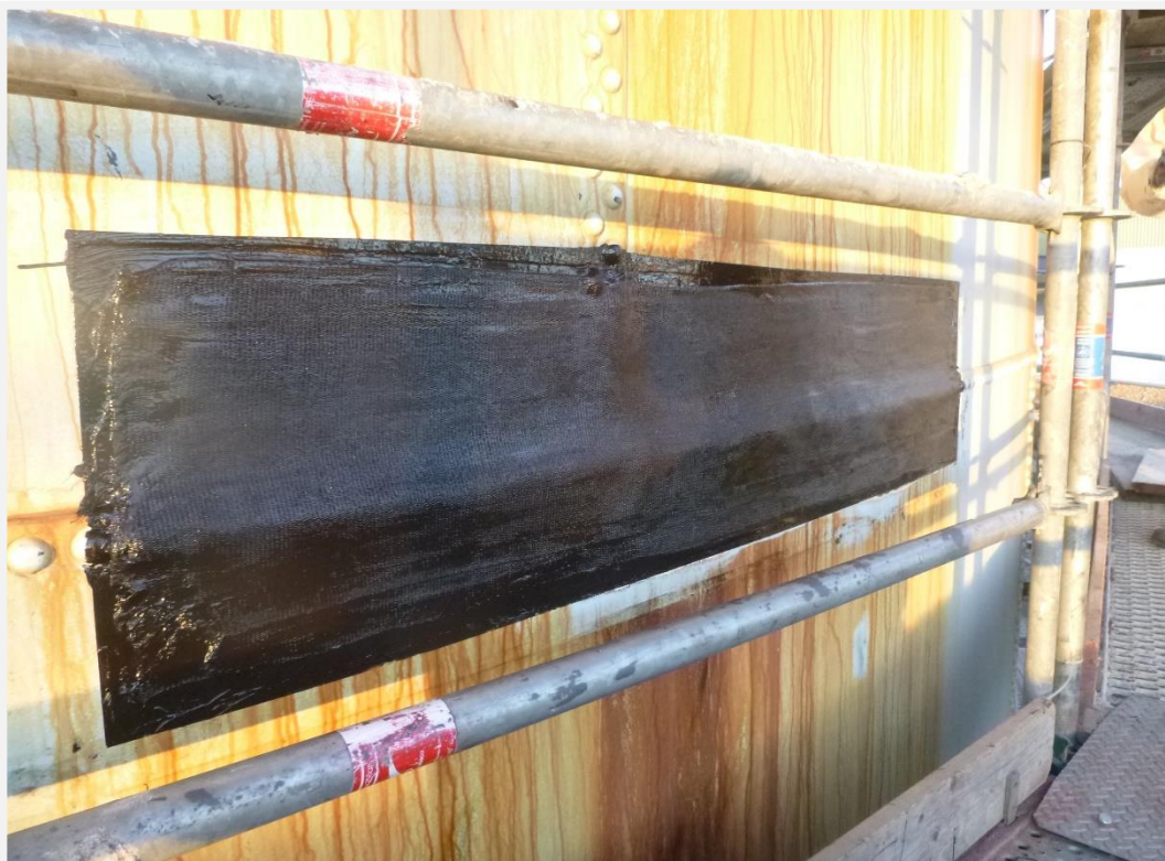
EXAMPLE OF PATCHING COMPLETED – AFTER REINFORCEKIT® PATCH
