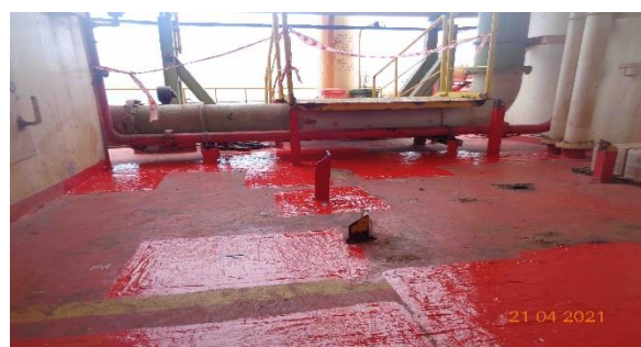
Fig. 8: Anti-UV painting applied
