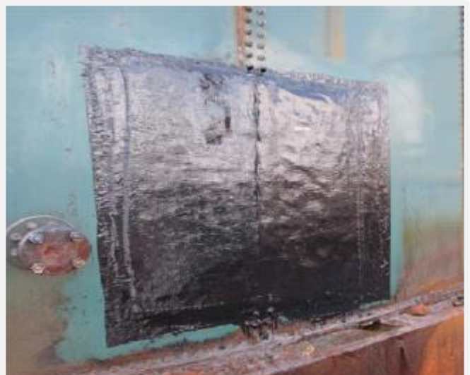
REINFORCEKIT® PATCH INSTALLED ON STORAGE OIL TANK (GABON) – BEFORE / AFTER
