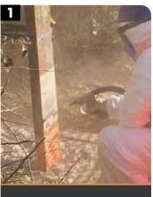
Surface preparation Sa21/2 / St3 and roughness Rz > 60 µm
