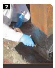
Epoxy resin application for corrosion protection
