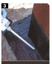
Waterproofing by elastomeric filler application
