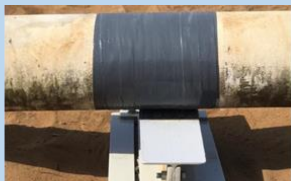
Fig. 5: View of R4D wrapping reinforcement in contact with ROLLERKiT product
