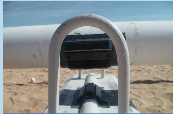
Figure 9: ROLLERKIT® installed on pipe and on support (configuration #1)
