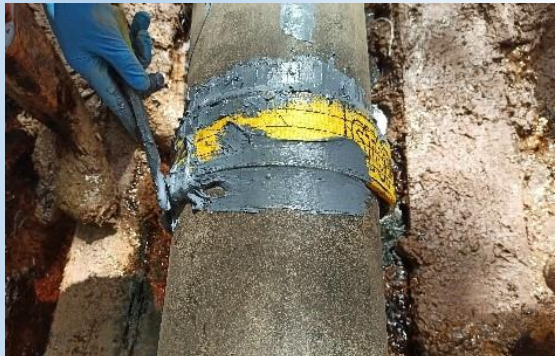
Figure 2: F3X8 filler application
