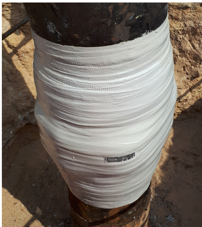
Figure 6. Reinforcement completed and identity plate installed for traceability.
