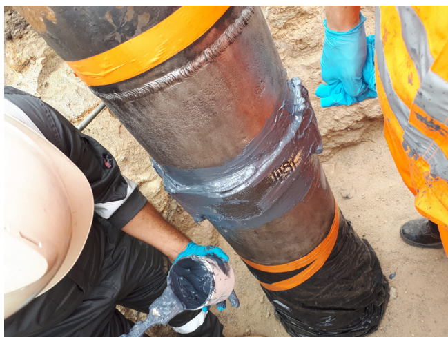
Figure 5. STOPKiT recovered with 3X filler before wrapping with R4D-HT+.
