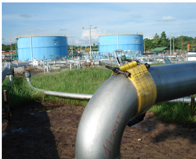
Figure 1. STOPKiT® product installed on an elbow.
