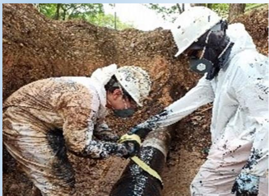
Figure 3: Composite wrapping on progress
