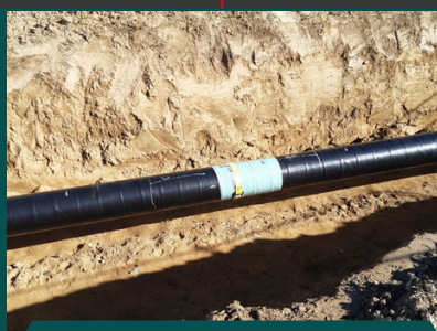
Fig. 5: Overview of the pipeline repaired with STOPKiT®
