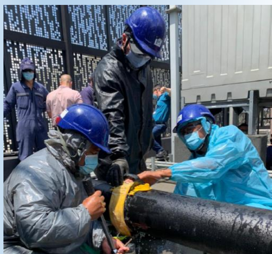
Fig. 3: STOPKIT® installation training on progress
