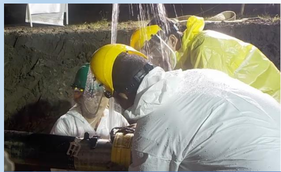
Figure 2: STOPKIT® positioning
