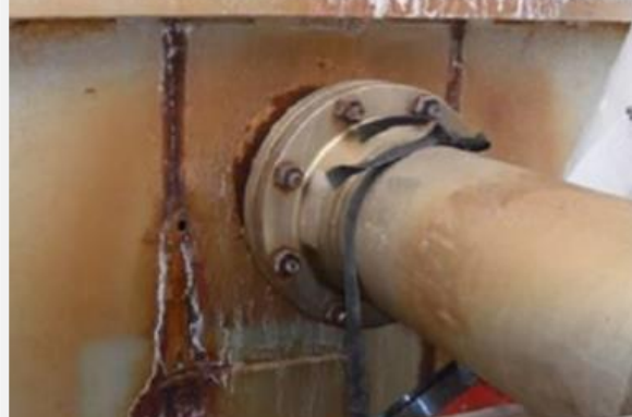
TANKIT PATCHING COMPLETED
