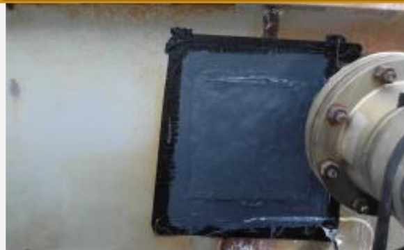
TANKIT PATCHING COMPLETED
